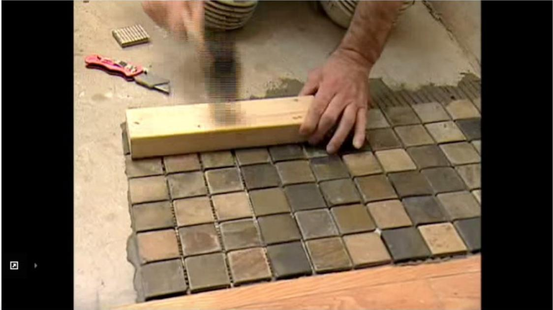
The video player shows a close-up of a person's hands using a yellow wooden straightedge to guide the placement of square mosaic tiles on a bathroom floor. The tiles are arranged in a grid pattern. A red-handled utility knife and a bucket are visible in the background.
